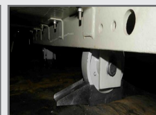
Roller anti vibration damper
